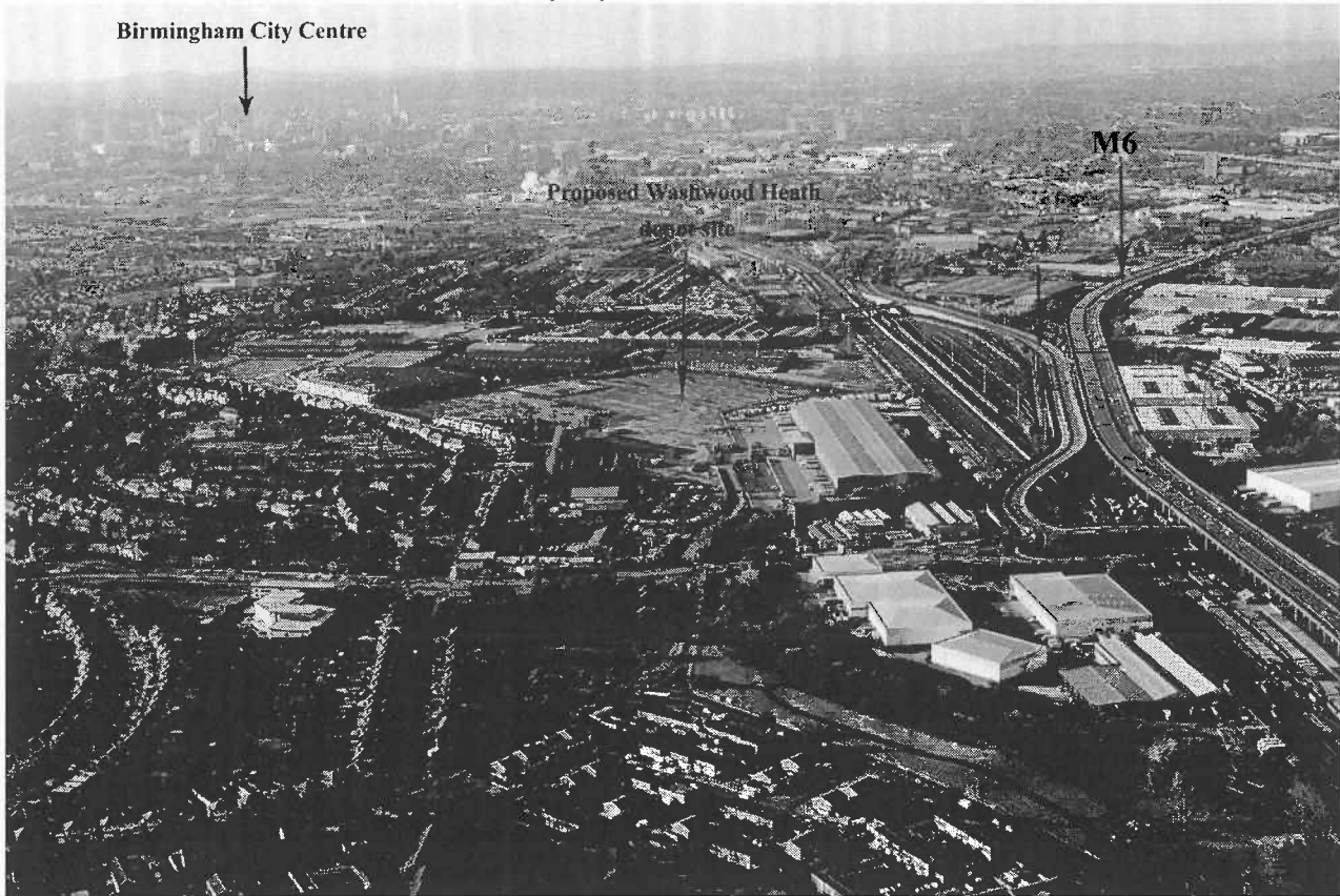
Aerial view of proposed Washwood Heath depot site [HS2 Ltd]
